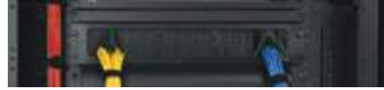
Brush strip models allow routing of cables through the panel.
