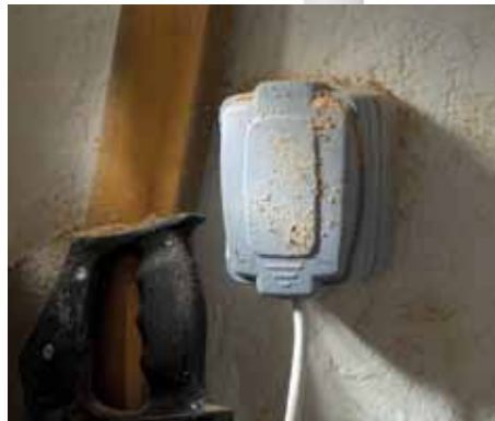
Dust proof connection to safeguard work areas.
