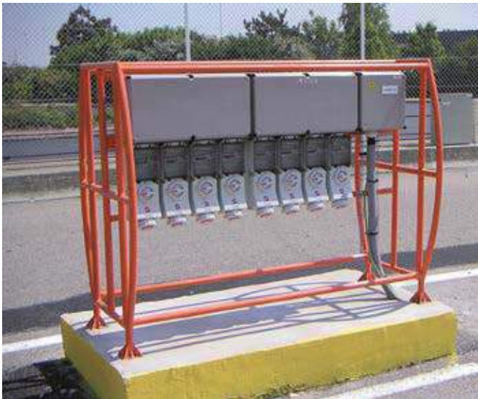
Container Terminal, Le Havre – France
